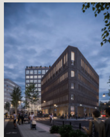
Ledvolten is an office building of about 4,500 m 2 . The building contains five floors and a basement. It will be built with commercial space on the ground floor and four flexible open office floors which the medtech company Carmeda has rented and will move into during the fourth quarter 2021.
